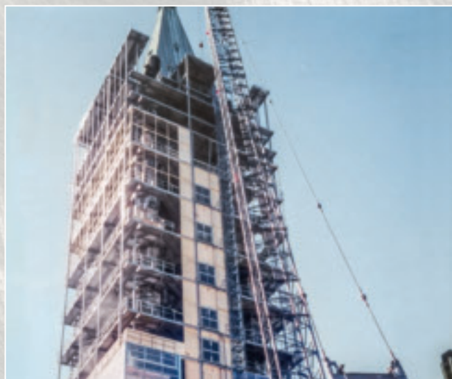
Peace Tower structural scaffolding system 1993.
