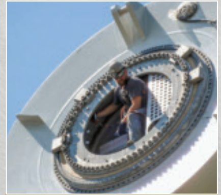
Local 700 apprentice Carl Lamoure, perched in the nacelle, is preparing to receive the rotor for connection.
