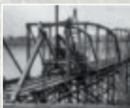
Erecting the Traffic Bridge in 1907.
