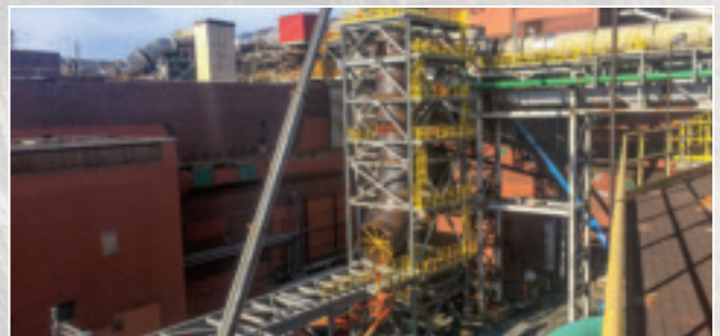
Ganotec, Supermetal and Local 786 erect new bag house and fan house at Vale's Clean AER project.
