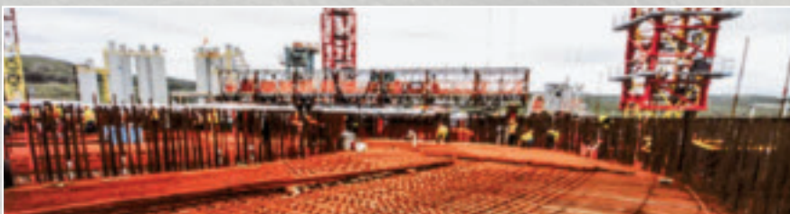
5,142 kilometres or 3,195 miles of rebar was used; if placed end to end it would go from Newfoundland to Vancouver Island and back, one-third of the way
