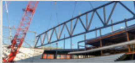
Impressive heavy truss of 223 feet long and 134,000 pounds was installed at Moncton Downtown Centre.
