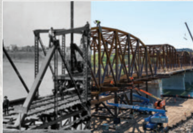
110-year time lapse of construction on the Traffic Bridge in Saskatoon.
