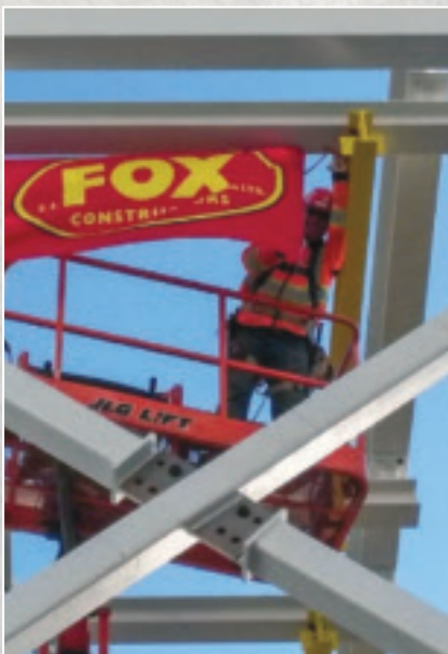
Robert Losee, Local 721, third-generation ironworker, placing the topping off banner for E.S. Fox Constructors Ltd. at the Retube Waste Storage Building at Darlington Nuclear Power Facility.
