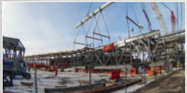
E.S. Fox and 786 install new converter flues and ducts.
