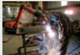
Protecting shop members during welding operations.
