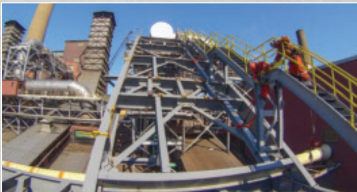
E.S. Fox and 786 install new converter flues and ducts.
