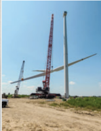
Crew is tailing the rotor section with all the blades pre-assembled on the ground.
