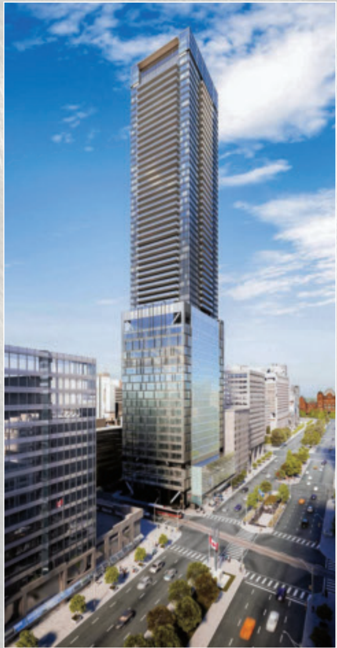
The 37 floors were erected to expand the existing 18-story office tower to 55 stories.
